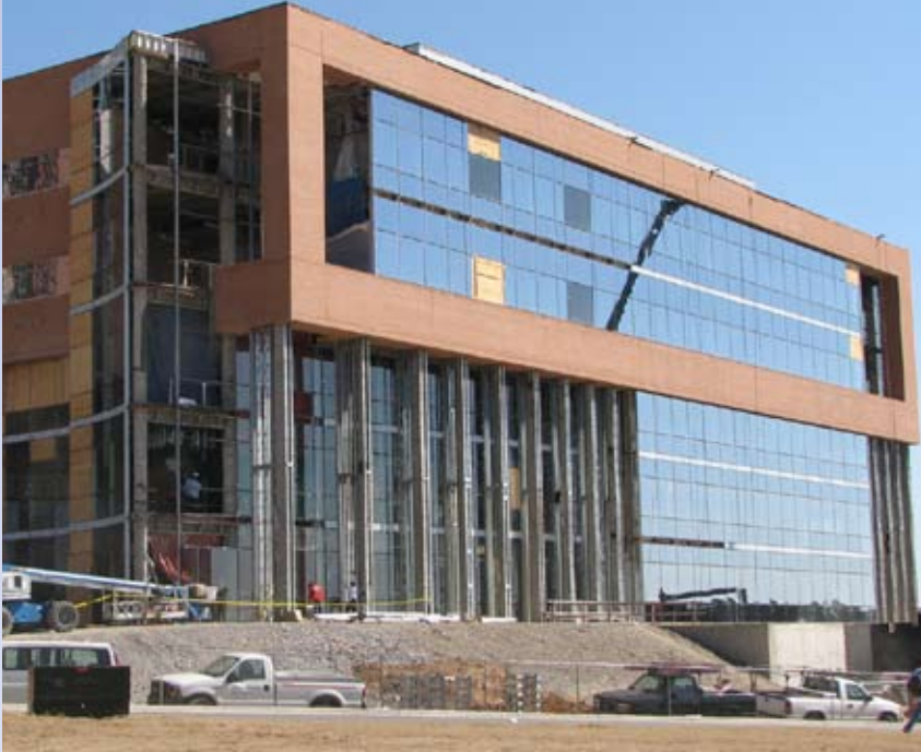
View of the west side of PRI as of March 12, 2008.
