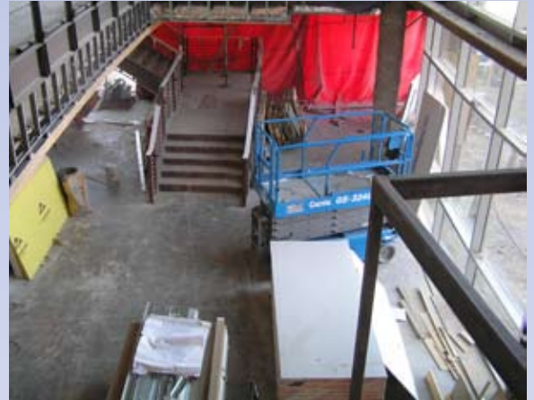
View from the second floor looking into the lobby.
