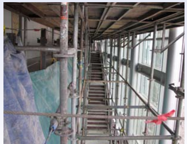
Monumental staircase in progress.
