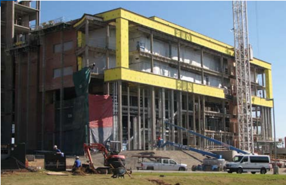
Progress on the PRI building as of November 12, 2007.
